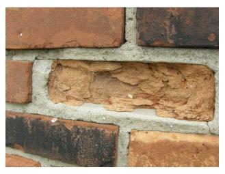
Spalling occurs when brick absorbs moisture, which expands in freezing temperatures, breaking apart the affected bricks. If bricks are painted, you may notice the paint flaking off. Using the wrong mortar mix can also be a cause. To avoid spalling:
